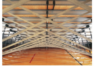
G. Tension Bracing Through bolted to the frame to provide additional stability. All bracing is coined to remove sharp edges, and all ends are rounded for safety.
